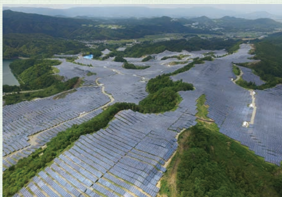
Matsusaka Solar Power Plant
