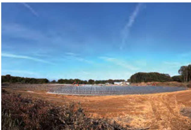
A solar farm under construction (Aomori Prefecture)
